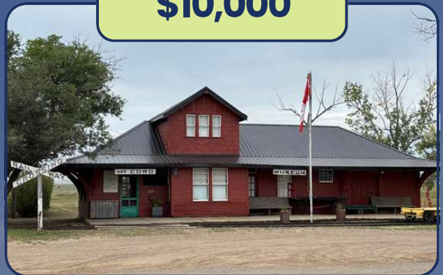
McCord Museum Roof Replacement
